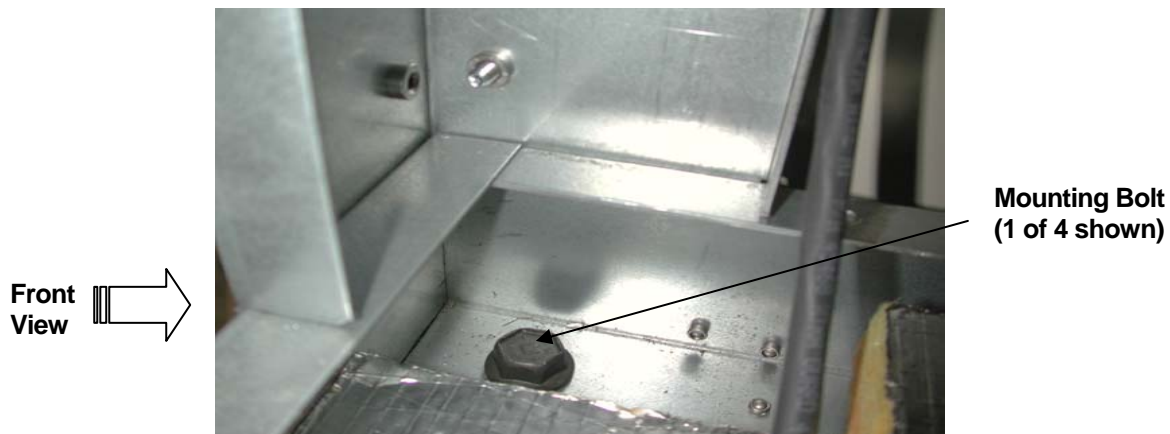
Figure 10. HRM Mounting Bolt Location
